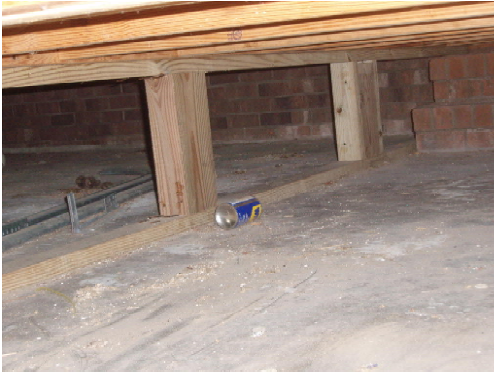
Foundation right room addition supports
